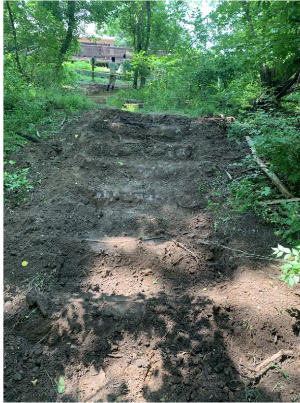
Step 2: Remove the old wooden steps and haul away.
