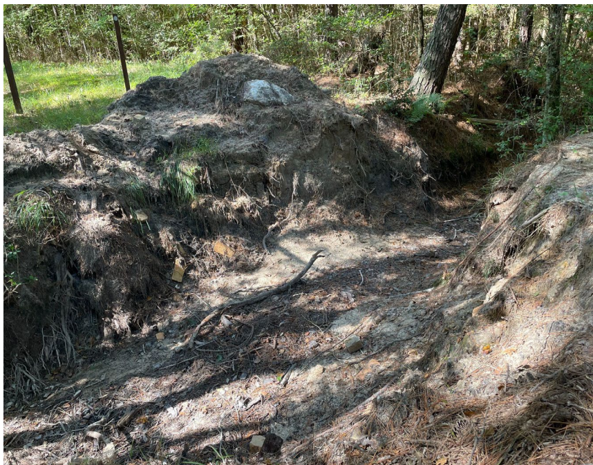
This shows how much erosion can occur when a water control structure is damaged.
