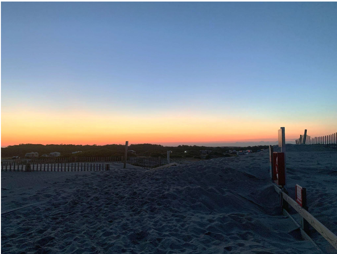
This picture shows sand covering the boardwalk at one of the campsite loops. Handrails are covered with sand and safety signs are nearly covered.
