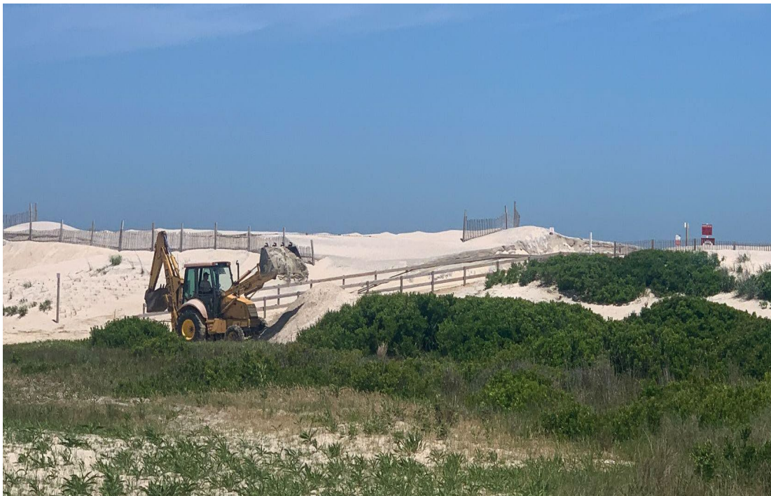
This shows a staff member removing sand from the dune crossing, an activity which is becoming more frequent.
