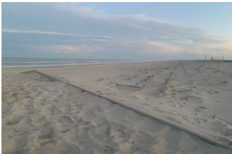
Sand covering the handrails on the dune crossing to the beach.
