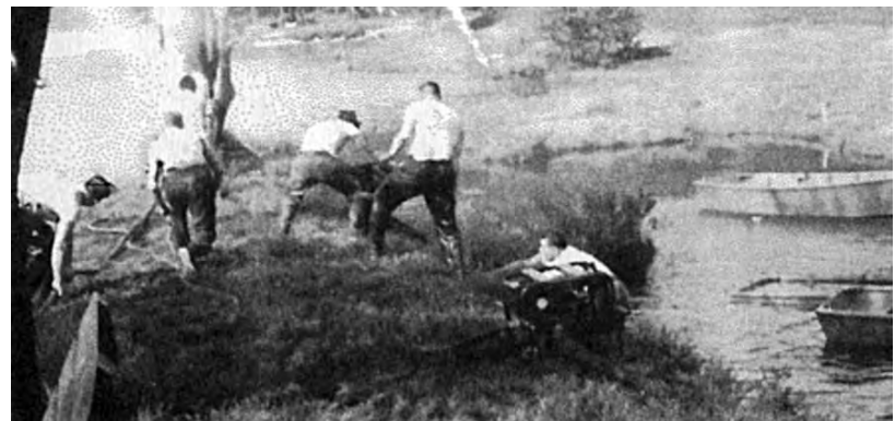
Fig. 34. Portable pump practice using water from Herrington Manor Lake.
